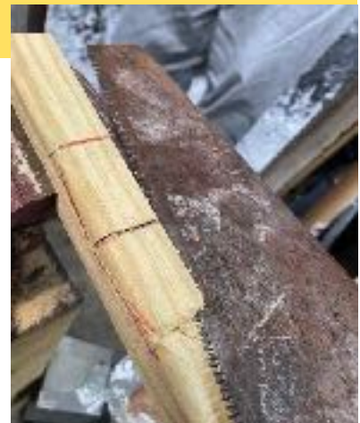
Figure 9: Hand saw the notch in the cross pieces.
