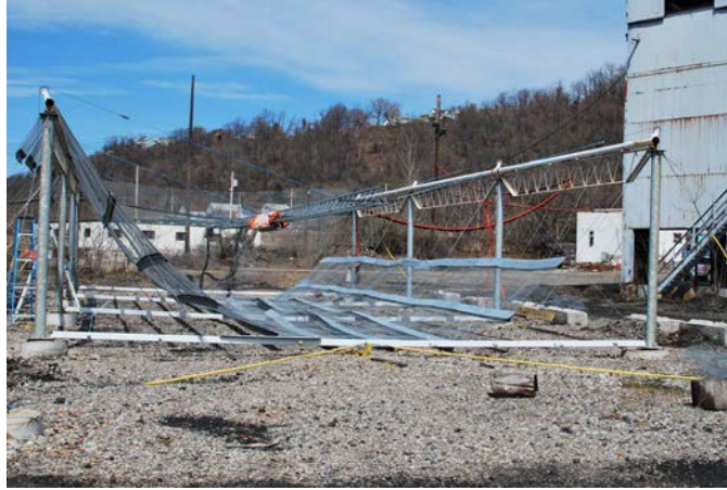
Figure 4.26: East cylinder re-attached and ready to raise.
