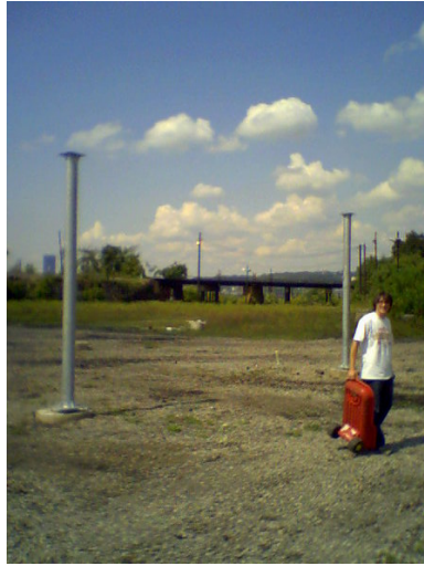
Figure 2.2: Putting up the columns. Wagon used to bring columns into place before raising. Columns were raised with just 2-3 people and no machinery.
