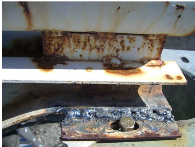
Figure 4.23: Finished weld
