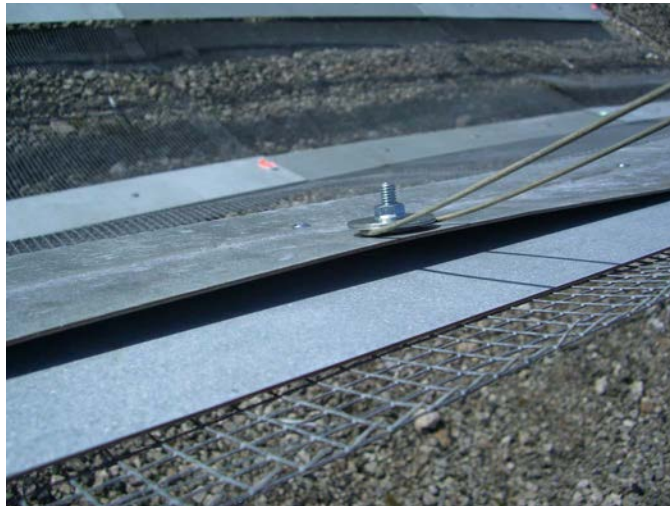
Figure 4.18: East cylinder new standard attachment of the mesh to the steel wire.
