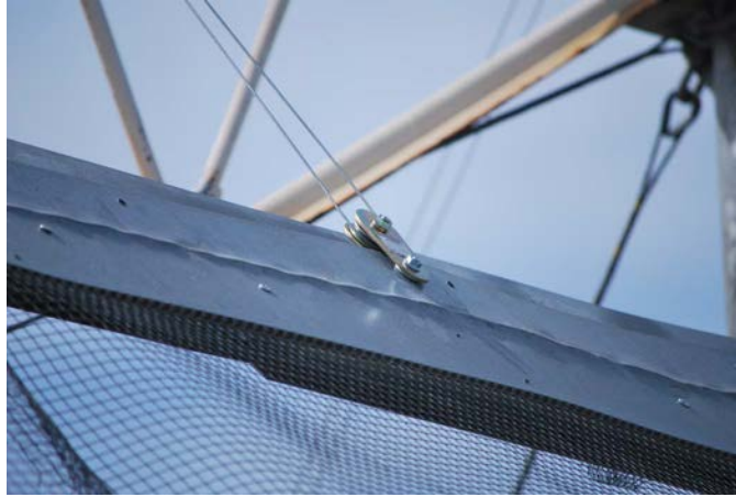
Figure 4.19: West cylinder new standard attachment of the mesh to the steel wire.
