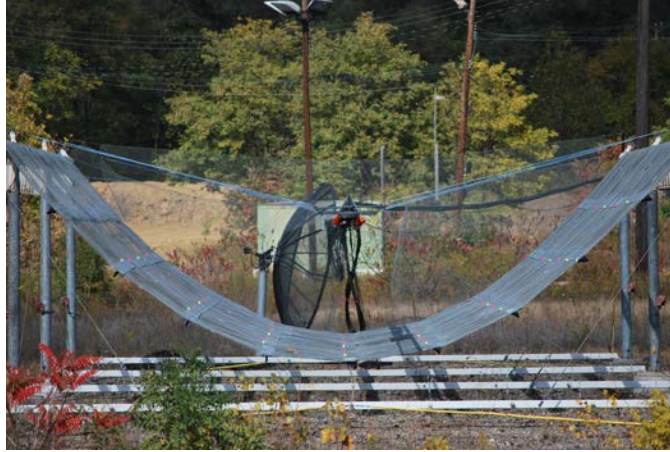
Figure 4.30: West cylinder raised and adjusted, mesh added back along the top side.
