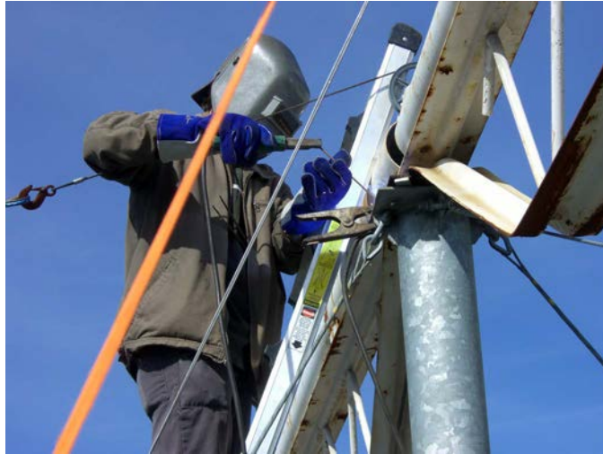
Figure 4.22: Welding the truss back together.
