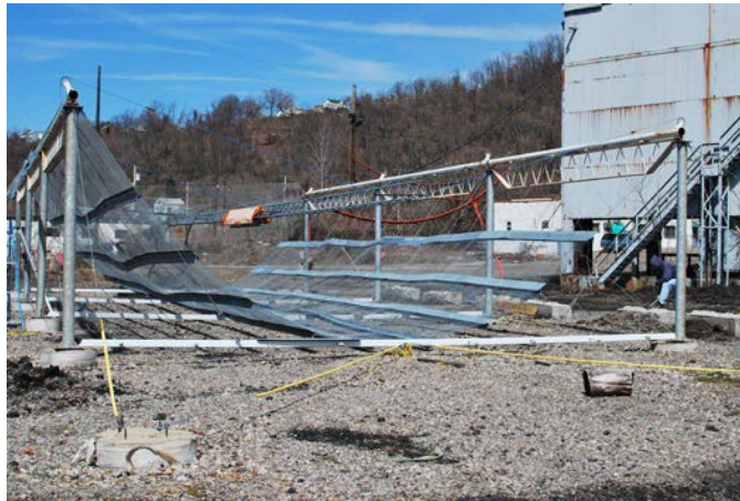
Figure 4.27: Raising the East cylinder. Each winch was tightened 10-20cm before moving to the next, going north-south along the cylinder.
