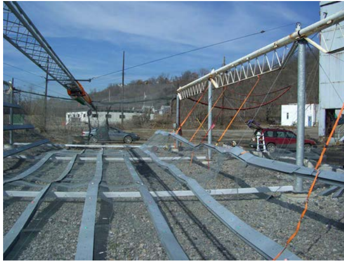
Figure 4.24: East cylinder at the start of the raising process. The top batten on the fallen side is brought to a working height with standard straps. Finger plates are attached to the mesh and steel wire, which then runs over the truss.
